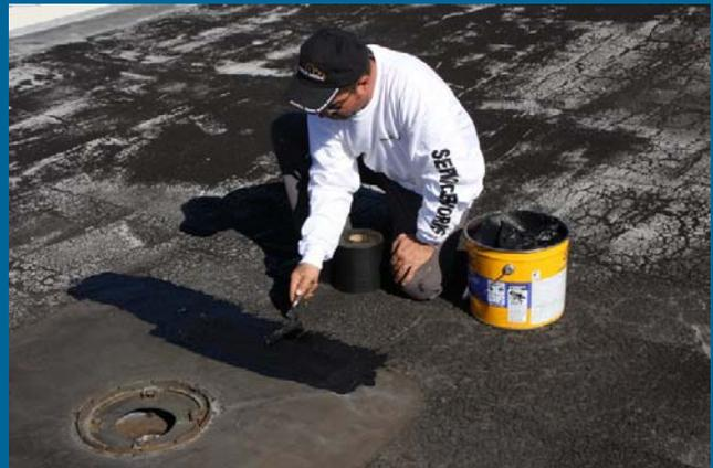
PVC, and Hypalon can be permanently repaired with a new piece of membrane heat welded to the cleaned roof surface. Duct tape can be an effective temporary patch for emergency situations. Self adhering patches work well provided that the adjacent membrane is thoroughly cleaned with detergent and wiped dry.
